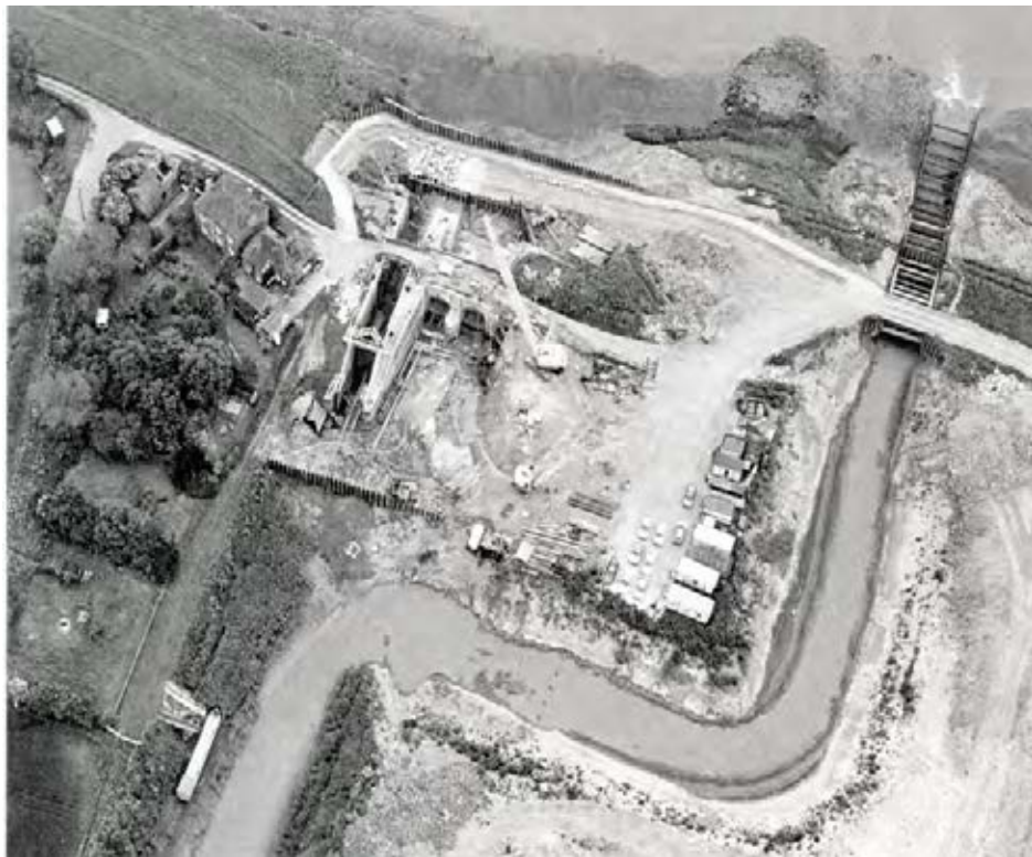
An Aerial View of the Lock Refurbishment showing the Diverted Canal
