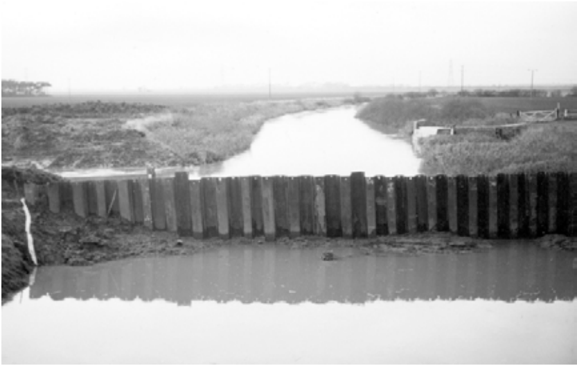
Temporary Cofferdam across the Canal
